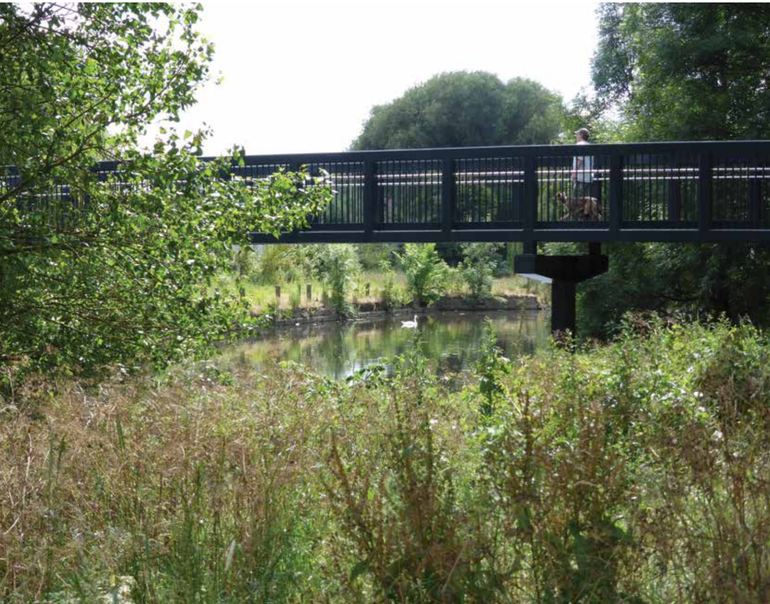
New bridge to improve access to the Dock development
